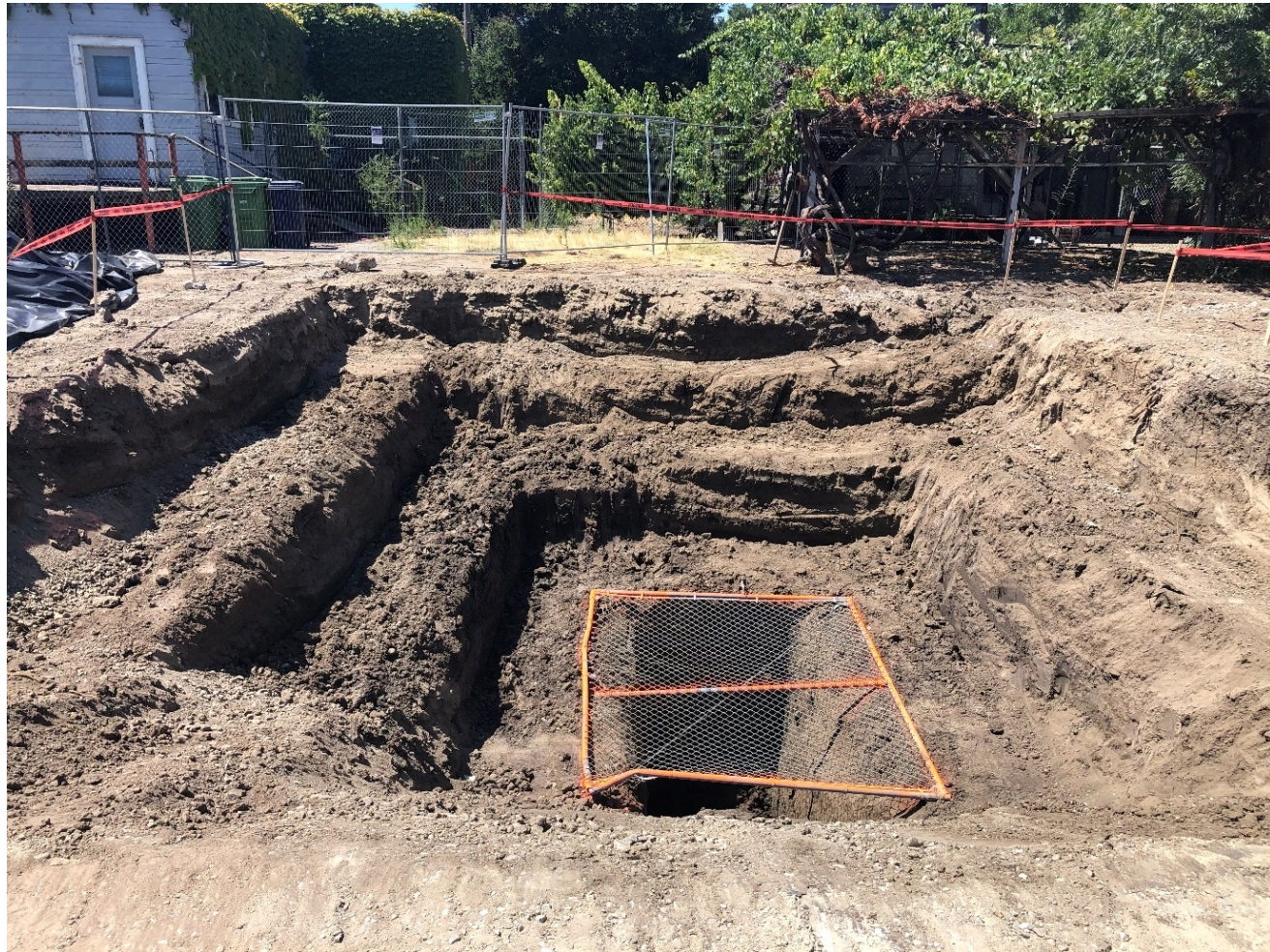
Borel Underground Storage Tank Removal
