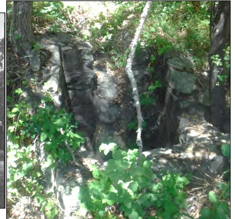
Overview of one example of ca. 1930 stonework (headwall) in Tilden resulting from Works Progress Administration/Civilian Conservation Corps work in Tilden. This type of stone culvert has been identified for Routine Maintenance (culvert) repairs and during Fuels work in Tilden.
